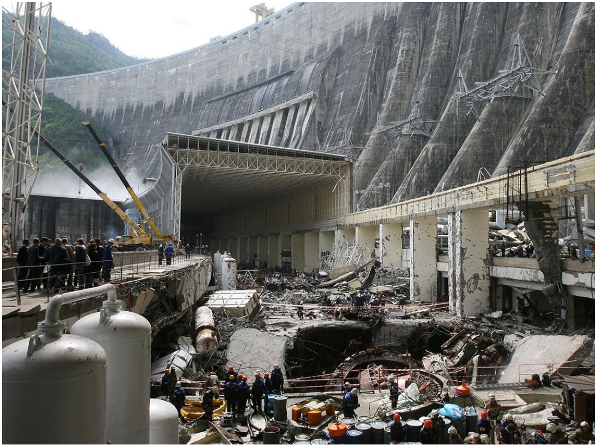
Fig. 4 – View of destroyed turbine hall at Sayano-Shushenskaya HPP after the disaster
